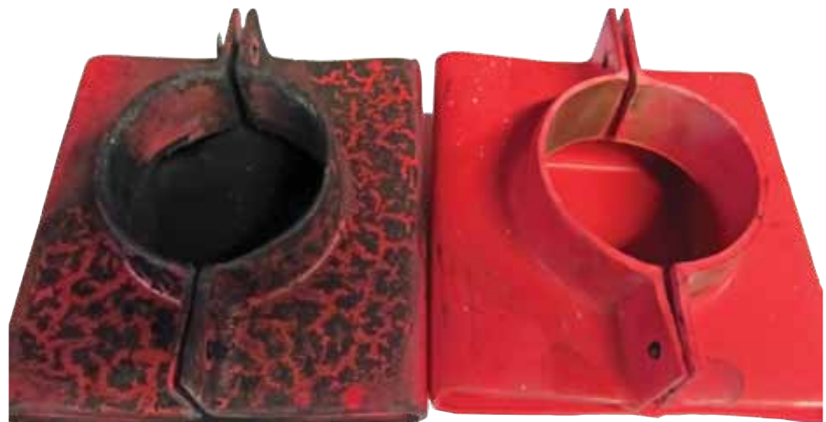
The associated bus joint boot shows the flashover damage.
