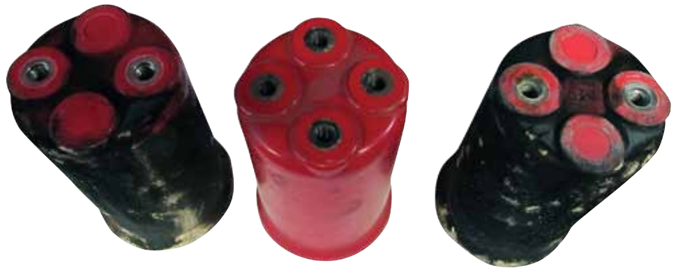
15-kV rated 6" Glastic insulator bushings with flashover damage resulting from a lack of switchgear inspection and regular maintenance. The center insulator is provided as a reference for what it should look like.
