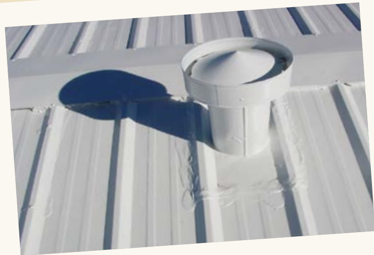
The sealed, finished roof.
