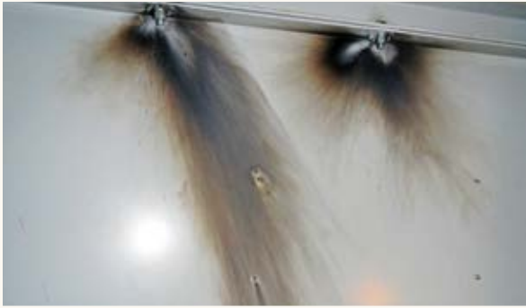
Evidence of arcing caused by faulty vacuum interrupter bottles.
