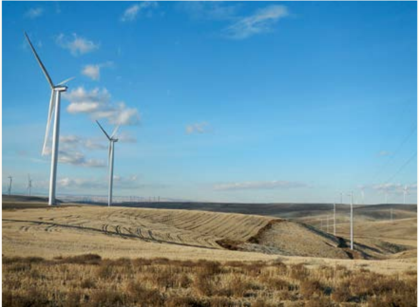
Vacuum Interrupters' third-generation magnetron atmospheric condition test system (MAC-TS4) enabled technicians to identify several new vacuum interrupters as the cause of periodic equipment failures at a major U.S. wind farm, potentially saving hundreds of thousands of dollars in equipment repairs and downtime costs.
