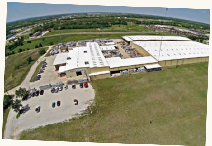
A Birdseye view of the CBS Gainesville Texas facility's new roof taken by kite using a GoPro camera.
