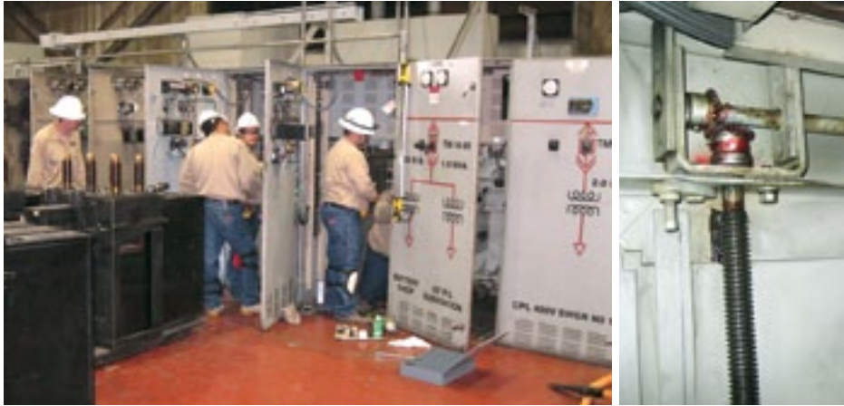
Left: WES's manufacturing capabilities were on full display when it rebuilt all cubicles for more than a dozen Magne-Blast circuit breakers for a U.S. steel manufacturer. Right: GE Magne-Blast AM 13.8-750-2H 2,000-amp with VCP-WR element air-magnetic circuit breaker that has been vacuum retrofitted.
