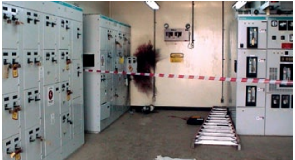
March 4, 2009, at the Jubail Project in Riyadh, Saudi Arabia: Three workers were removing a 480-V, molded-case circuit breaker from the bucket of an energized motor-control center (MCC) when an electrical arc flash occurred, severely injuring them. All three sustained first- and second-degree burns and were hospitalized following the accident. Myth: Switchgear is designed with arc-flash containment in mind.
