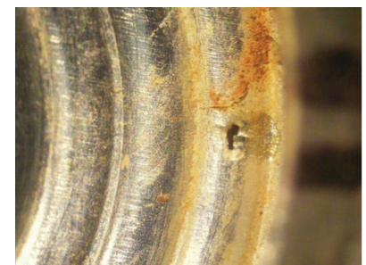
Figure 1. Galvanic corrosion in stainless steel bellows.
