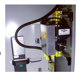
When accompanied by a CBS ArcSafe remote switch operator (RSO) control unit, the RRS-3 reduces the need for arcflash suits and eliminates all hazardous manual contact with gear during operation from up to 300 feet away. The system is lightweight and portable for hard-to-access areas.
