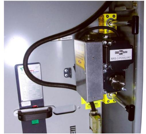
When accompanied by a CBS ArcSafe remote switch operator (RSO) control unit, the RRS-3 reduces the need for arc-flash suits and eliminates all hazardous manual contact with gear during operation from up to 300 feet away. The system is lightweight and portable for hard-to-access areas.
